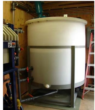
**Figure 2 – Reactor Tank & Mixer**
