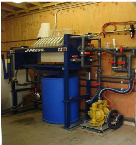
**Figure 4 – Filter & Transfer Pump**
